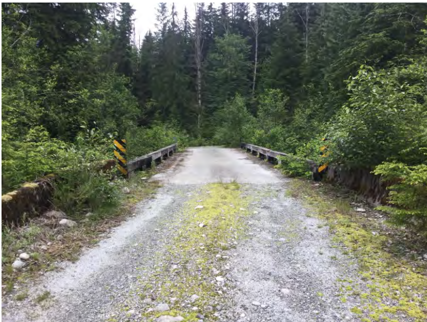
Approach from Left Bank when facing downstream
