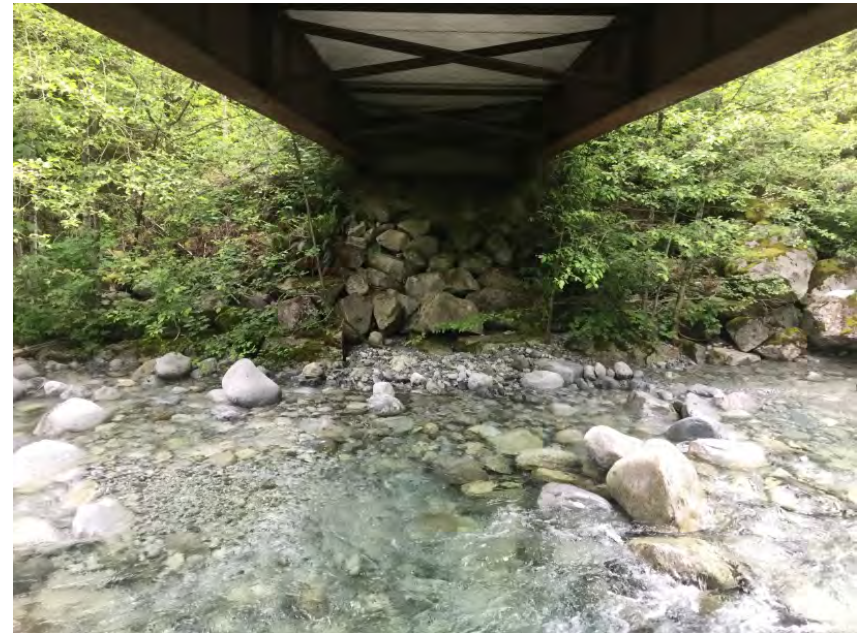
Right Bank Abutment when facing downstream
