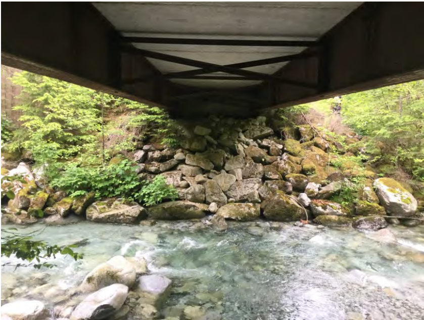
Left Bank Abutment when facing downstream
