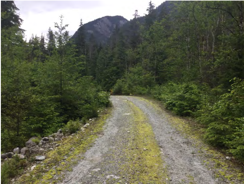
Approach from Left Bank when facing downstream
